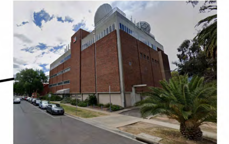
Communications Building 4 Storeys
