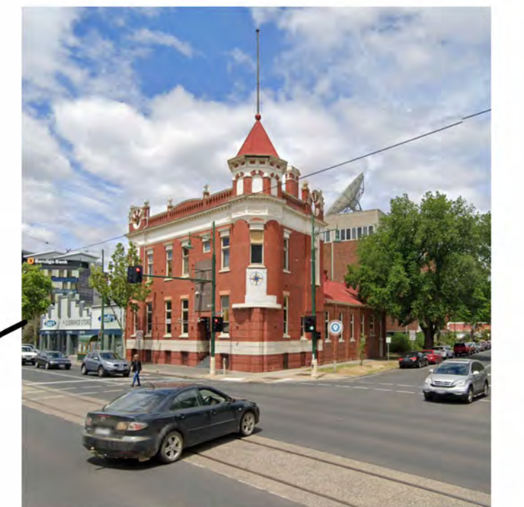
Previously YMCA Building 3 Storeys
